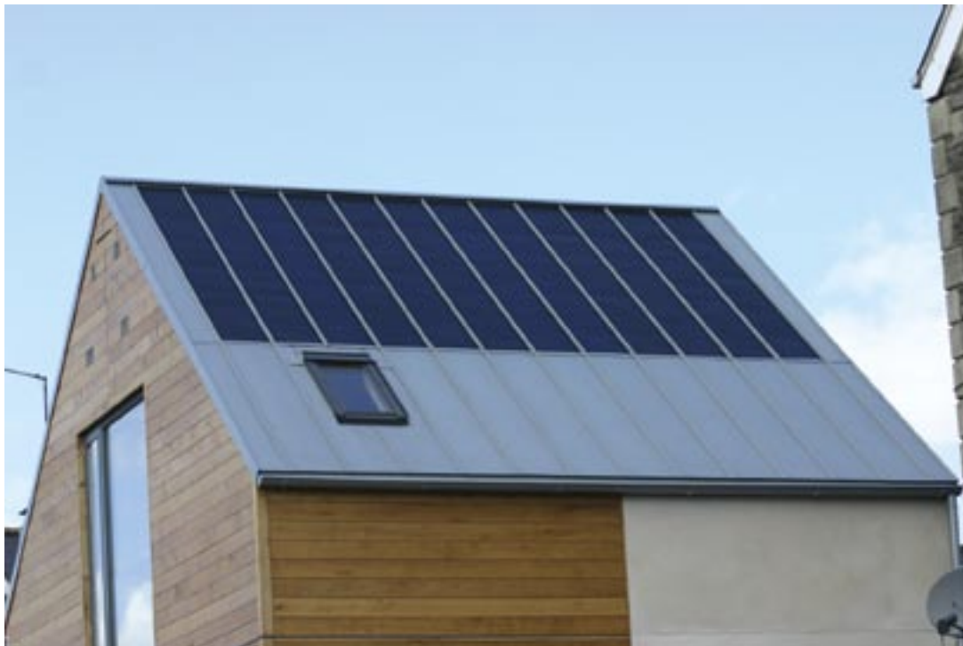
21 | Solar panels, Coach House, Cardiff
