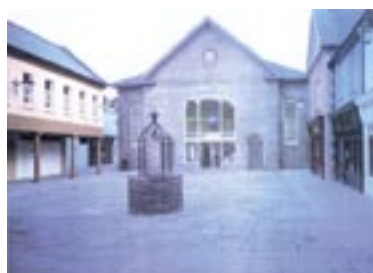
25 Listed Buildings at Bethel Square, Brecon
