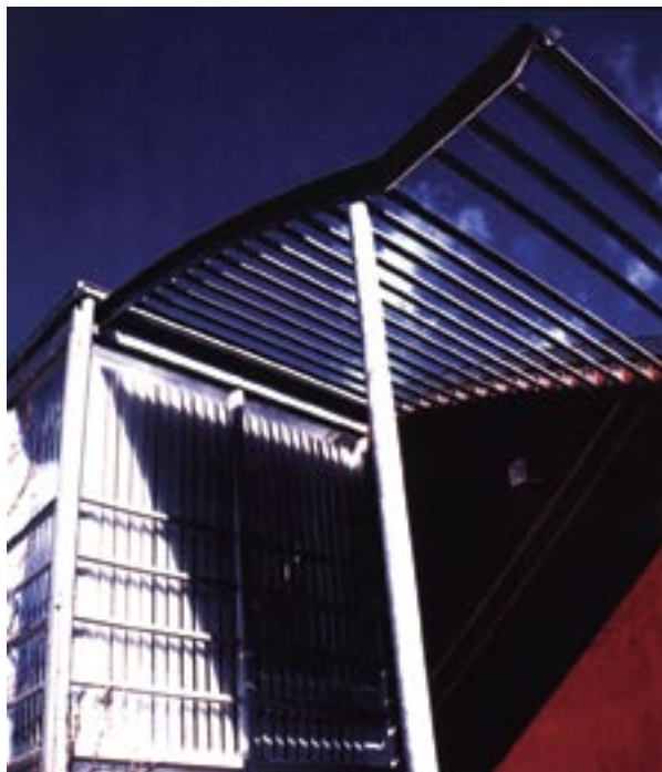
16 | Solar shading in SA1, Swansea
