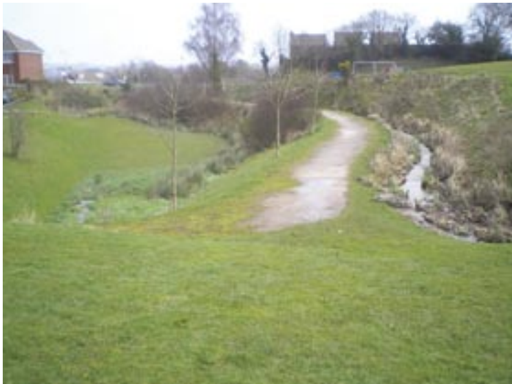
39 Sustainable drainage systems at Pontyclun
