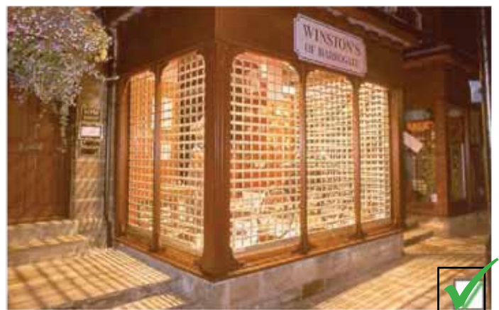
Internal perforated roller shutters behind the external glass provide adequate security and still allow for window shopping and encourage activity outside opening hours.
