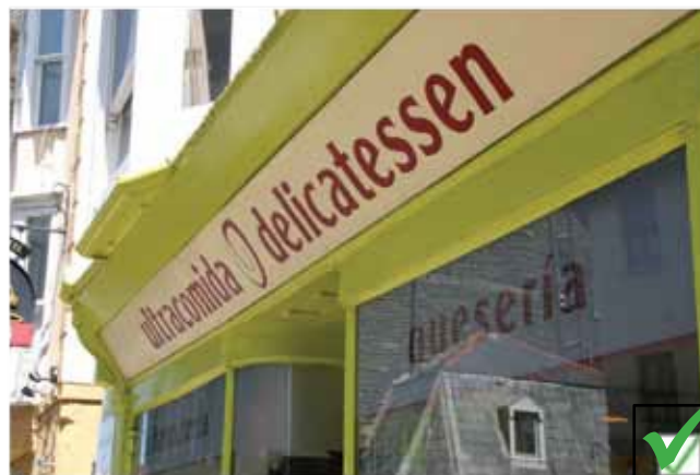
Fascia is in proportion and ties in with the shopfront as a whole.
