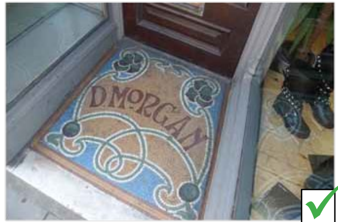
Use of terrazzo flooring and other tilework can be a way of reinstating original features or adding new unique elements
