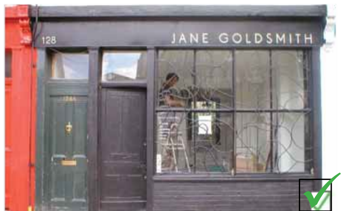
Decorative latticework behind the glass becomes an attractive and permanent feature of the shopfront.
