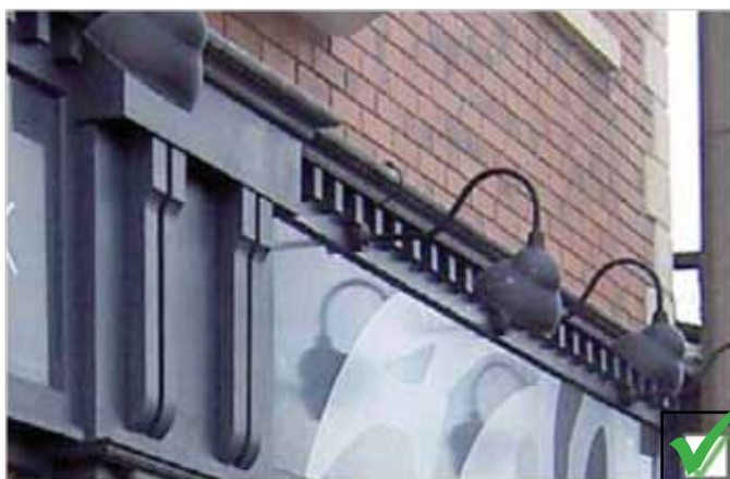
Externally mounted lighting fixtures are likely to work better on traditional shopfronts
