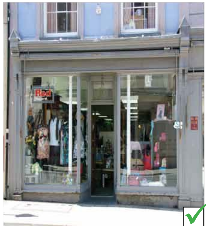
Pilasters (and to a lesser degree mullions) perform an important role in framing the shopfront
