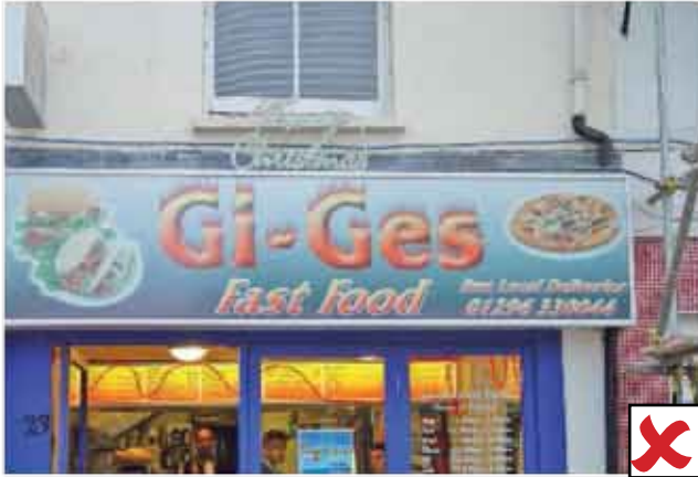
Oversized fascia prevents any chance of the shopfront relating to the rest of the building as a whole.
