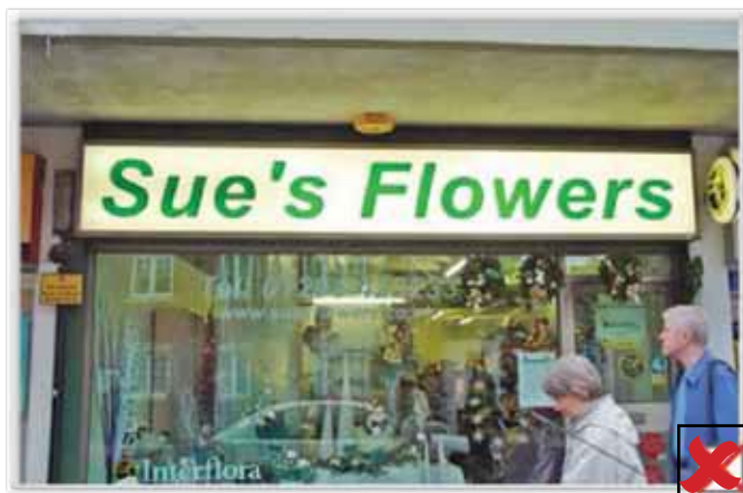
Back illuminated box signage appears crude and unbalanced because it dominates the shopfront. Furthermore it is not an integral part of the shopfront but an 'addition to' the shopfront
