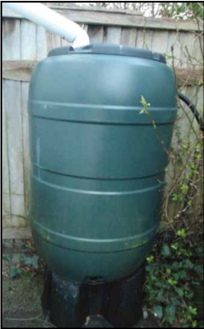
Figure 7.1 A garden rainwater butt.
