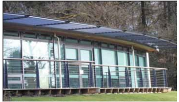
Figure 4.7 Brise soleil incorporated into the design of the Woodland Resource Centre, Cyfarthfa Park.
