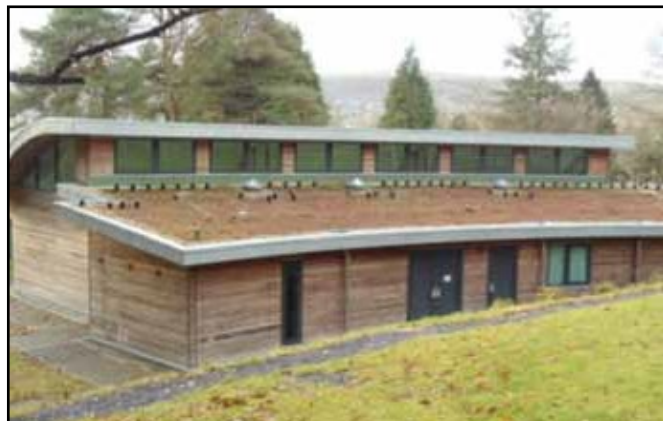
Figure 10.1 Green roof incorporated into the design of the Woodland Resource Centre, Cyfarthfa Park.
