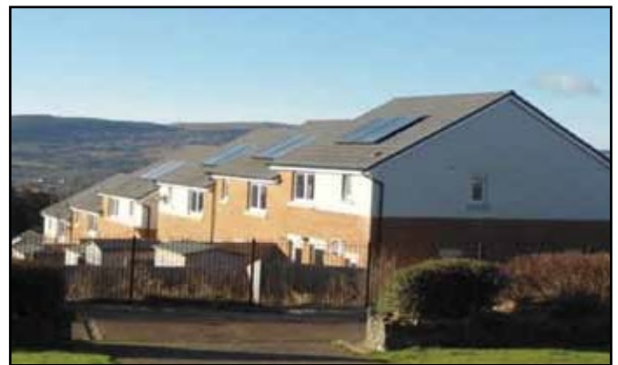
Figure 5.1 Roof mounted solar thermal panels on residential dwellings at Glanmor Gardens, Dowlais.
