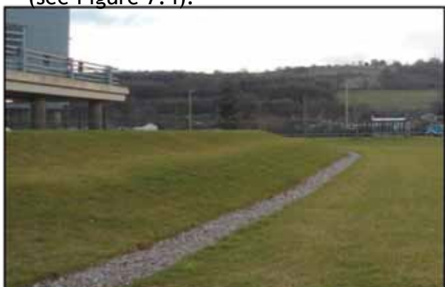
Figure 7.4 An infiltration trench incorporated into open space within the grounds of a hospital.
