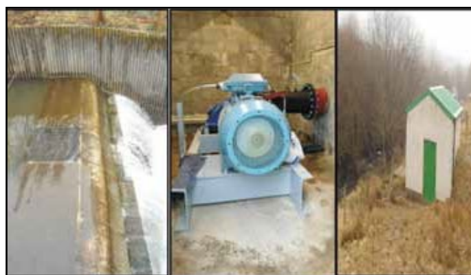
Figure 5.3 Micro hydropower scheme with a 26 kW power output providing electricity to the Blaenavon World Heritage Centre. Photos include the water intake (left), turbine generator (centre) and generator building (right).
