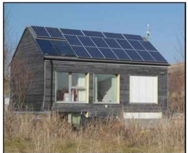
Figure 4.8 Externally mounted blinds providing solar shading on the Larch House, the Works Site, Ebbw Vale.
