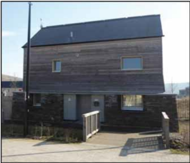
Figure 8.1 Pembrokehire larch cladding used on the Larch House, the Works Site, Ebbw Vale.
