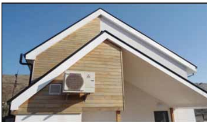
Figure 5.2 Air source heat pump attached to the side elevation of a house.
